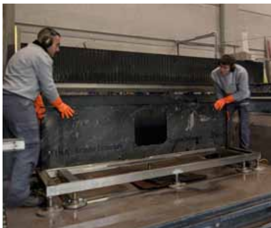
Corte y pulido del fregadero Sink cutting and polishing
